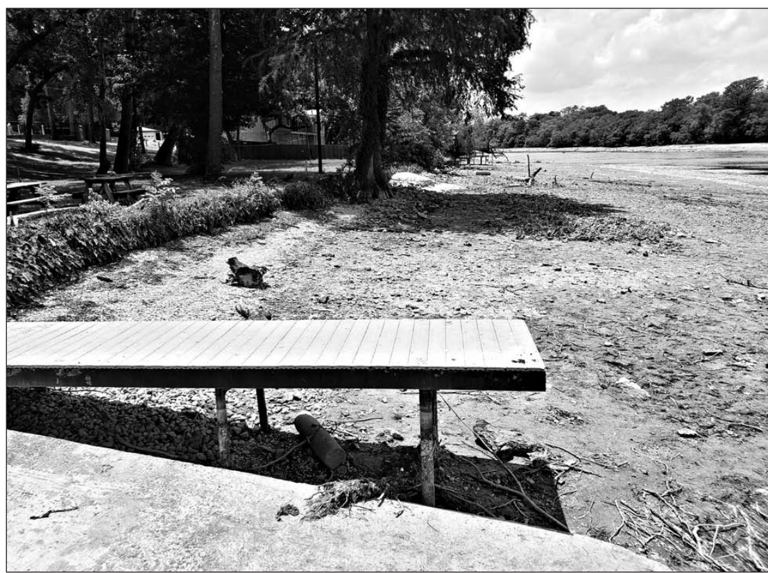
A DRY-GULCHED RIVER CHANNEL is all that remains of Lake Dunlap after a severe breach in the dam drained the Guadalupe River lake. (Photo courtesy of Guadalupe-Blanco River Authority)
